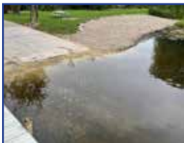
Embankment improvements at Villa Grove
